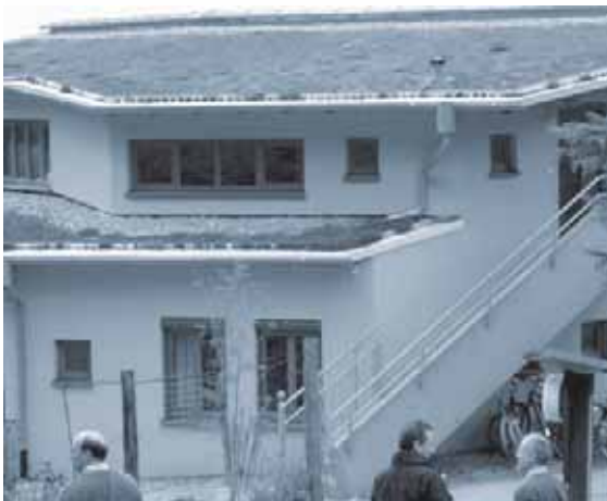
Extension building with extensively planted roof, retention value 50%
